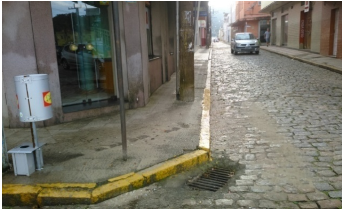
Figure 10: Intersection House at Gustavo Richard Street and Tenente Bessa Street, art deco exemplary. Source: Claudione Medeiros, 2015.
