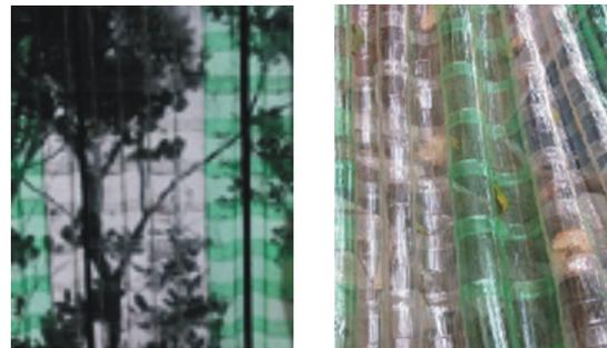
Figure 12: Eaves Coverings using Polyethylene Bottles. (Author's design)
