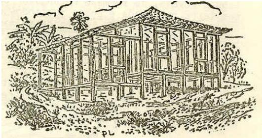
Figure 13: Frame for a Colonial House made ready to receive Wattle and Daub. Source: Revista Projeto, n. 28. p.75.
